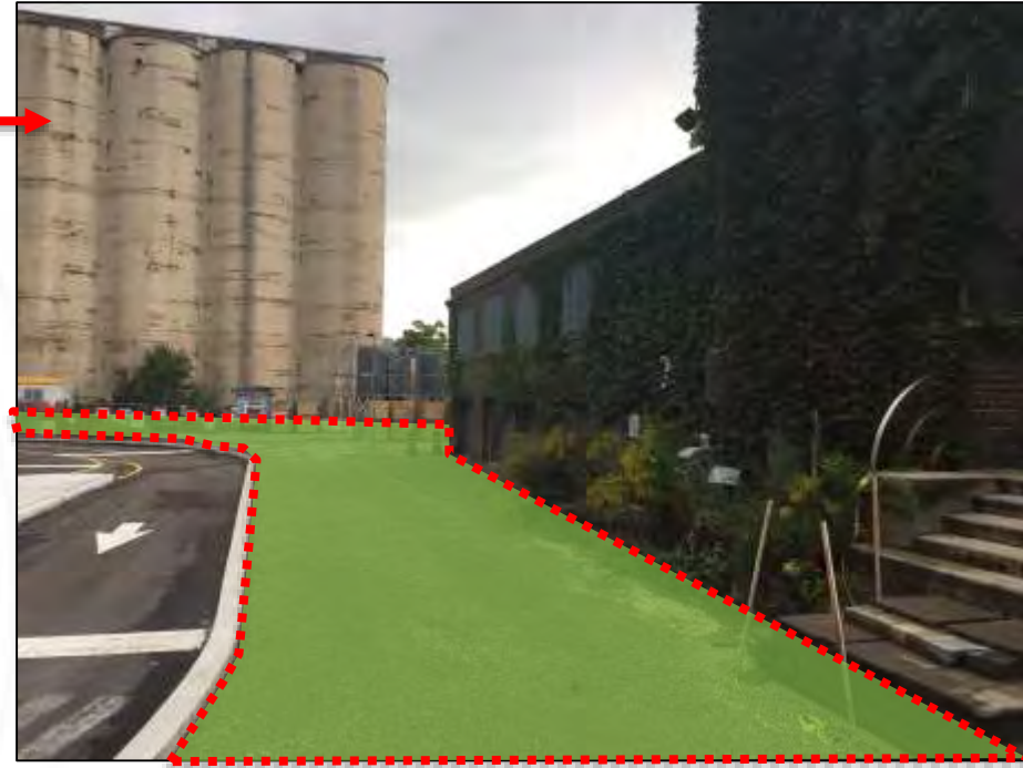
(Right) In progress: new pedestrian connection to Ireland Park
