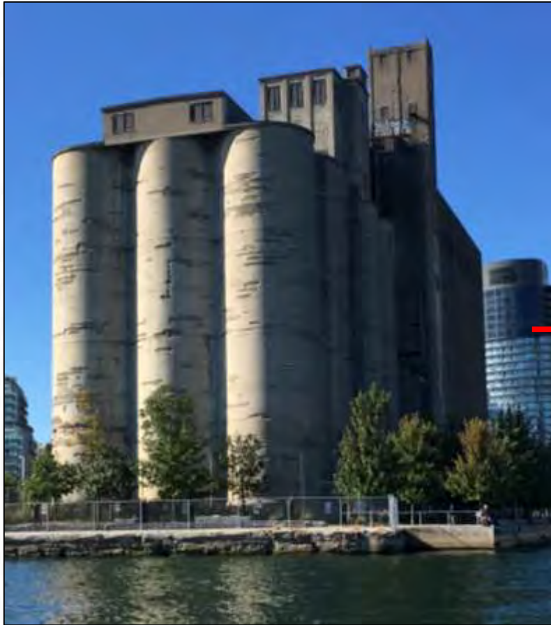
Before: dockwall deck was structurally compromised
