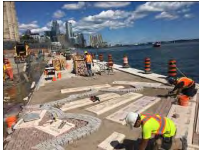
Granite cobblestone installation now underway
