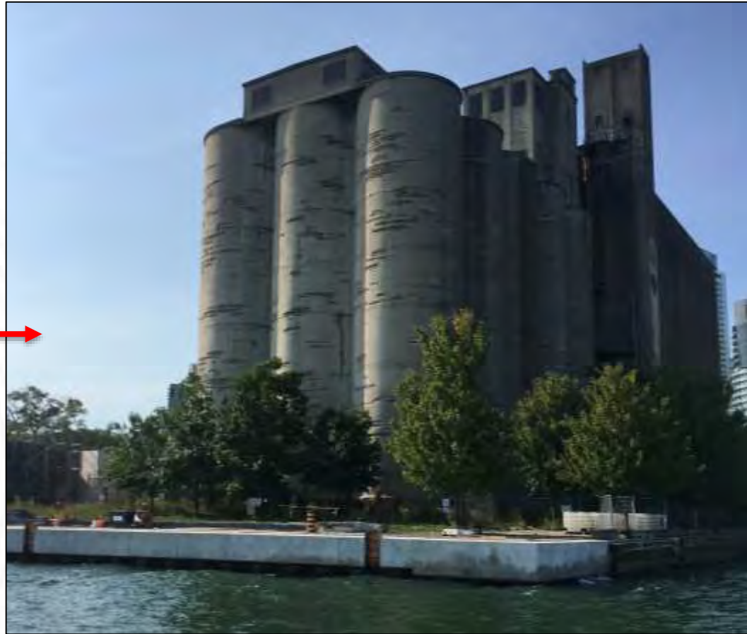
After: dockwall structural rehabilitation completed
