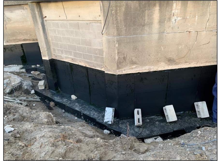
Above: Foundation waterproofing presently underway. Below: Hydro duct bank installation set to commence.
