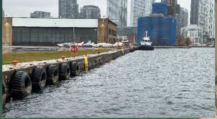
Island East Dockwall Rehabilitation
