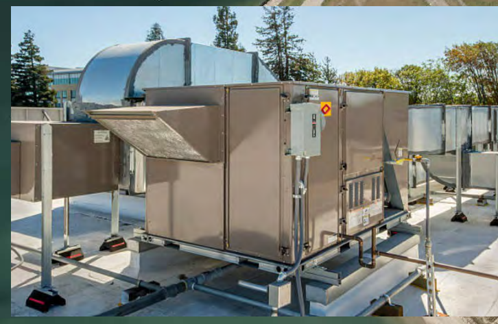
Climate Control Unit Replacement at Mainland and Island PTF's
