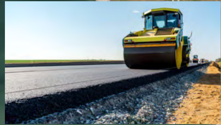
West Service Road Rehabilitation
