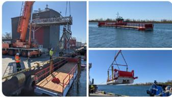
While the original steel supports and handrails were in good condition and able to be salvaged, the bridge floats and wooden decking were heavily deteriorated and needed to be replaced as part of this rehabilitation project. To ensure its longevity and structural integrity, the entire bridge was re-welded, sandblasted and epoxy coated, and a new wooden decking for the pedestrian crossing, built of Douglas fir, was installed.
