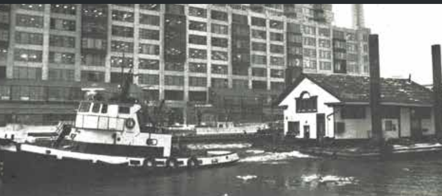
Above: Pier 6 was rolled onto a barge in 1988 and towed across Toronto Harbour for storage while work was carried out on a new foundation.
