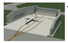
The GRE's steel framed structure is fully lined with acoustic panels designed specifically for the purpose of absorbing engine sound and reducing noise on the surrounding community. Through a design-build analysis it was determined that an optimized orientation would be at 250 degrees.
