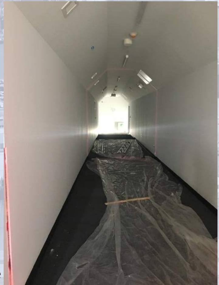
Interior of Module Temporary Gate
