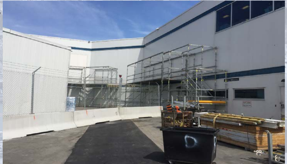
Covered access walkway erection on West Side
