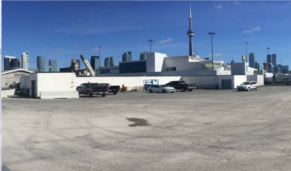
Completed Temporary gates exterior (Gate 3A)
