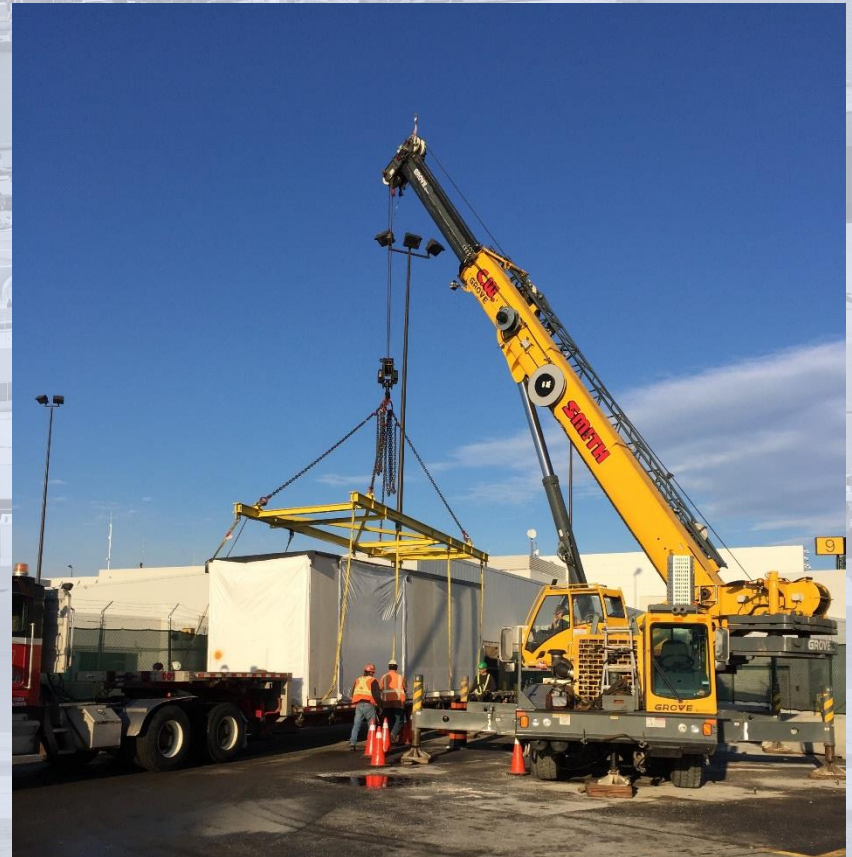
Module Temporary Gate 8A and 8B Installation
