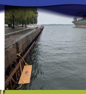
The duckling docks are wooden platforms, 12-inches wide and six-feet long, attached to an existing floating dock or dock wall. Each dock is equipped with a beveled edge to make it easier for ducklings to climb aboard.
